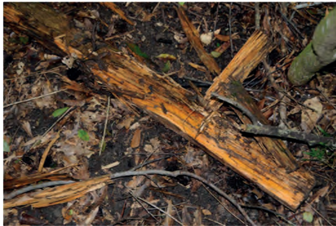
Figure 6. Randomly placed feeder stakes around the test site were completely consumed by Formosan termites.
