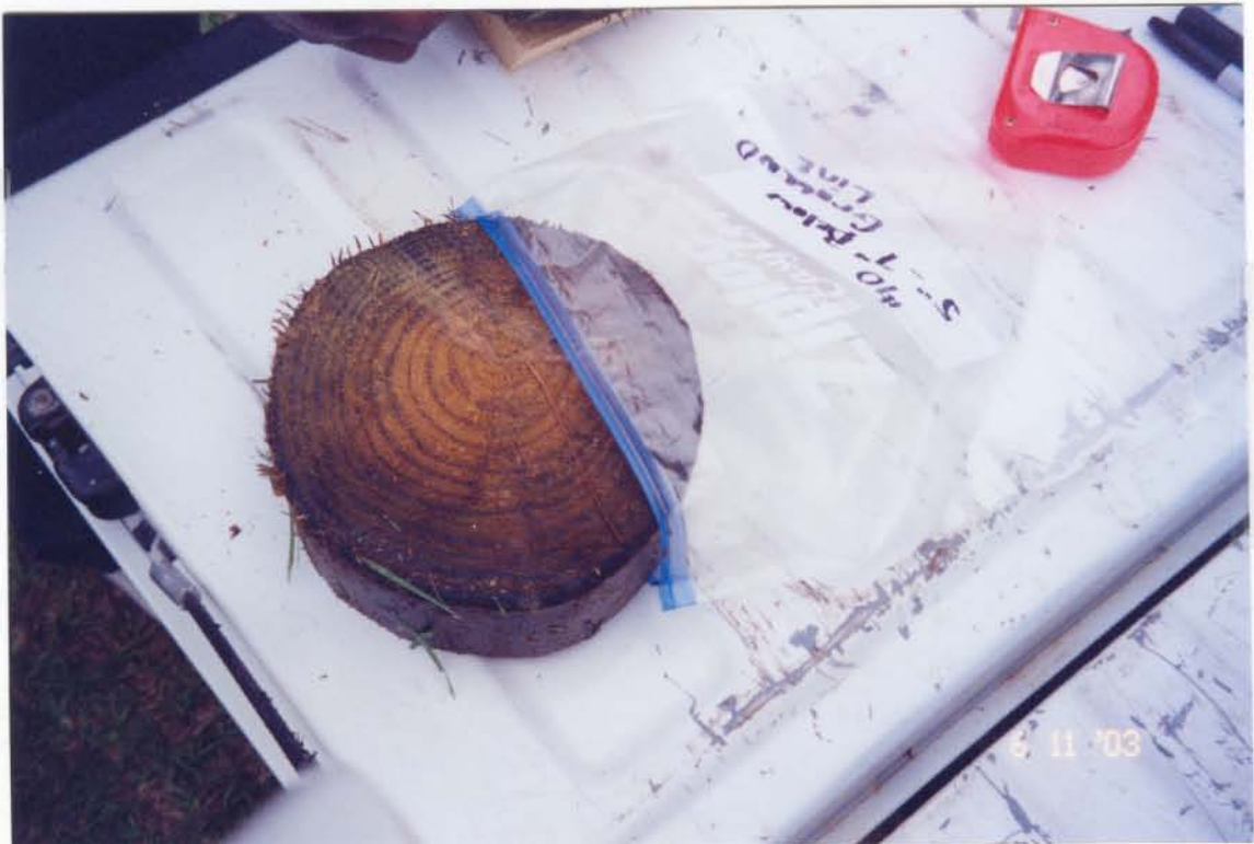
POST #10 5" to 7" below groundline
